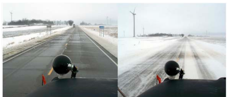
Segments of roads with living snow fences (left) have better driver visibility and road surface conditions than those without (right), leading to lower road maintenance costs and fewer accidents. Courtesy of the University of Minnesota © 2011
