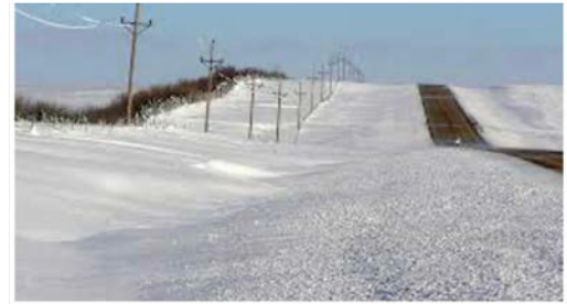
Orientation, length, height and density are all factors that determine the efficacy of a living snow fence to capture and store the greatest amount of snow.
